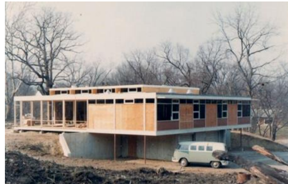
The Garber House under construction
