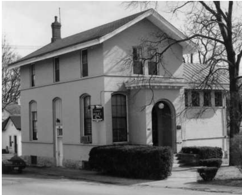
Glendale Police Station (1975)
