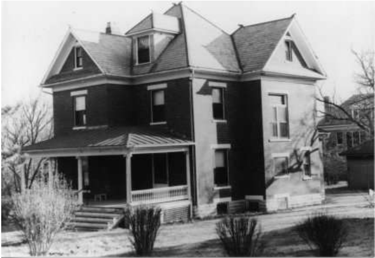
Home demolished by Cincinnati Bell.
