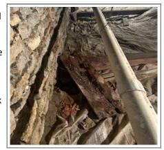
have been left behind when the building was built in 1880. In addition to the lumber, old pipes and the deteriorated vapor barrier that had covered the dirt floor in an attempt to control the moisture also had to be removed.
